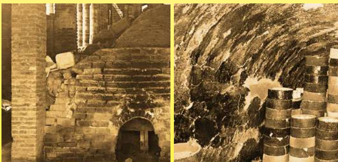
Traditional Chinese Dragon oven (龙窑 Long Yao), feeding mouth and filling method with electric porcelains (private collection)
